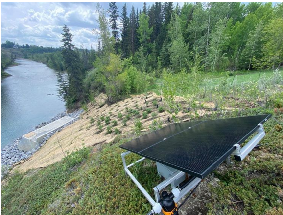
A solar-powered irrigation system at a riparian restoration site along the Elbow River in Calgary (Credit: Leaf Ninjas)
