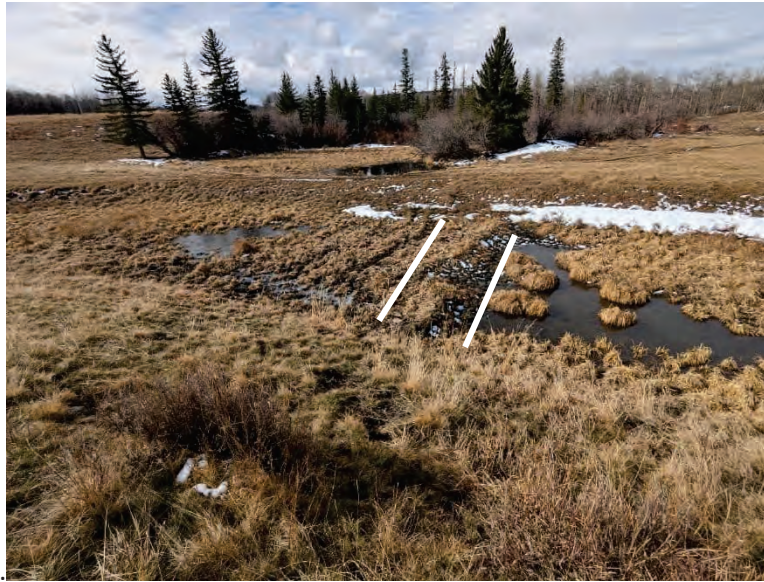
Figure 1: Grassed Weir at Sta. 0+050 Backing Up Water
